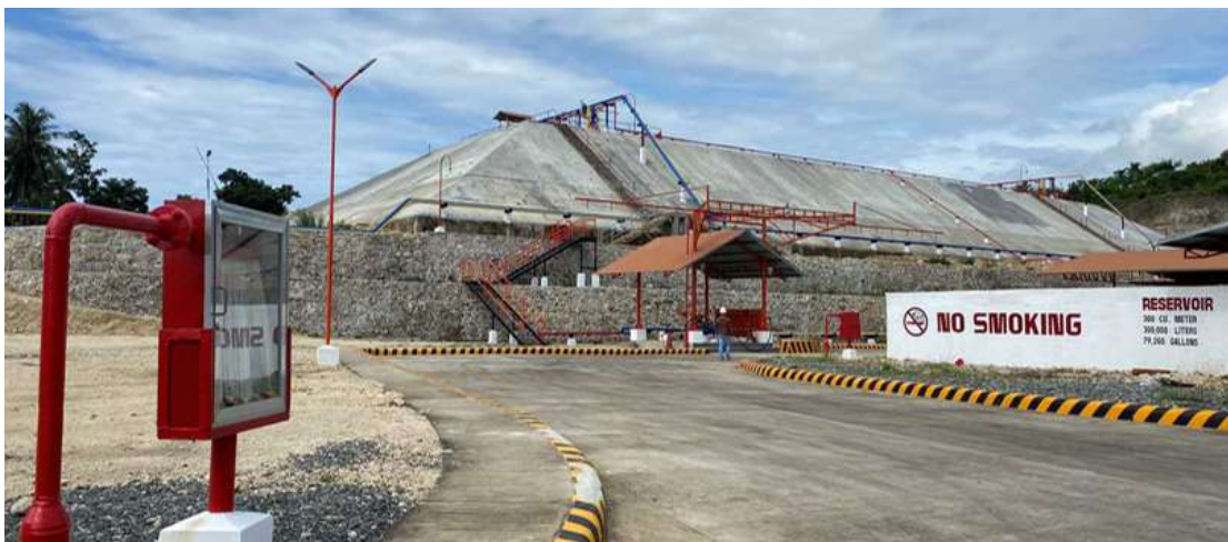
MOUNDED PRESSURE VESSEL TANK
